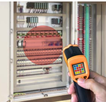
Transformers & distribution boards
